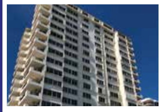
2. Project: Florida Tower Condos Location: Miami Beach, FL 19 story building
