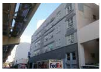
1. Project: Leamington Hotel Location: Miami, FL Over 80 Rooms
