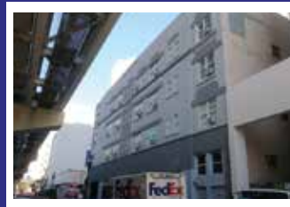
3. Project: Leamington Hotel Location: Miami, FL Over 80 Rooms
