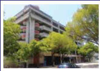
1. Project: Hickman Garage Location: Miami, FL Over 1,000 Parking Spaces
